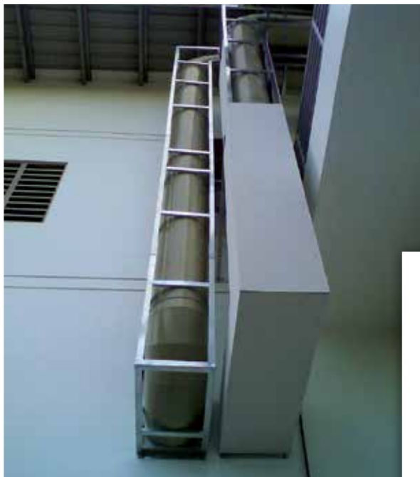
General M&E services enclosure at the carpark of Tseung Kwan O residential building in Sai Kung District, New Territories, Hong Kong (above) and outside the warehouse of 9 Benoi Sector, Singapore (left). Both use PROMATECT®-H boards.
