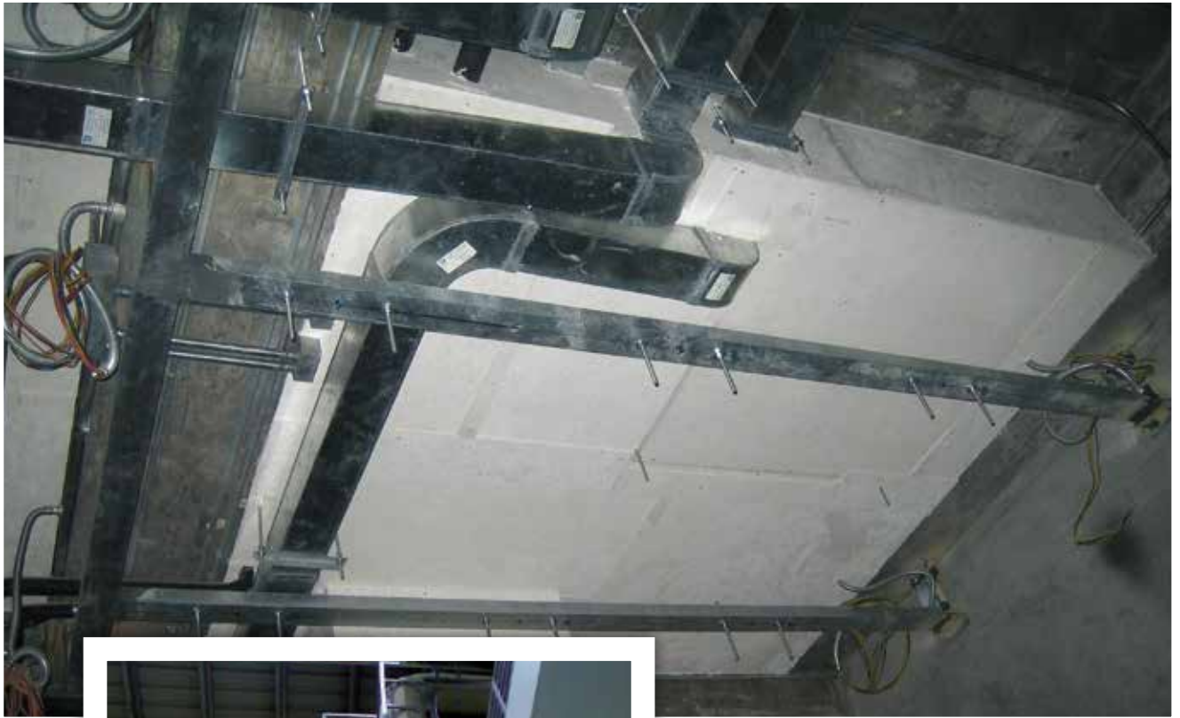
General M&E services enclosure at the carpark of Tseung Kwan O residential building in Sai Kung District, New Territories, Hong Kong (above) and outside the warehouse of 9 Benoi Sector, Singapore (left). Both use PROMATECT®-H boards.
