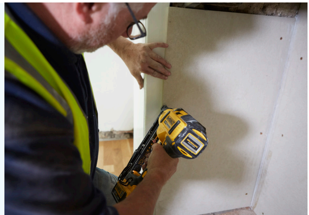
Fixing using a nail gun.
