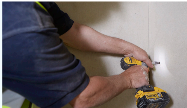
Screw being loosely fixed to the rear board.
