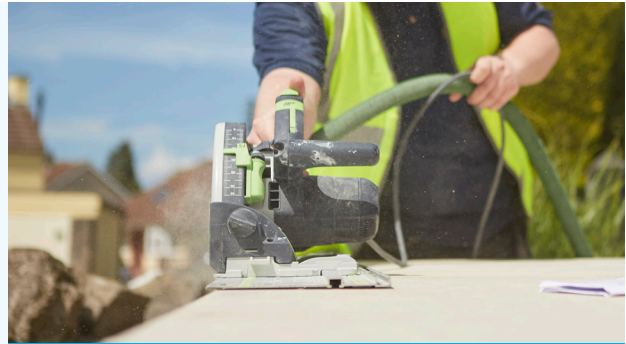
Using a Festool Plunge saw to cut.
