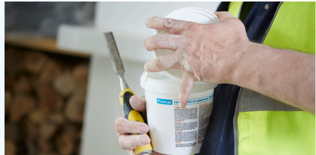
PROMAFOUR®-HT Joint Filler is applied to fill the screw heads.
