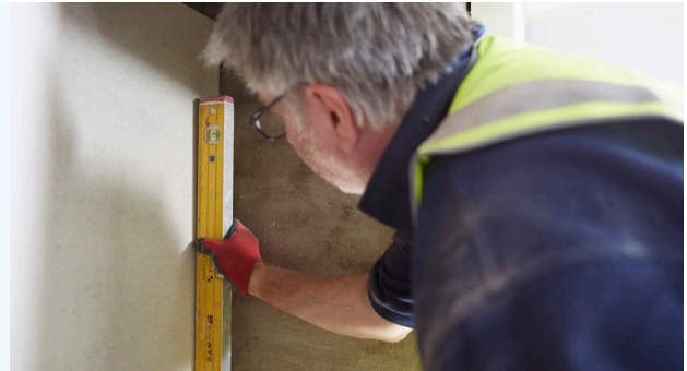
Checking the board is level.
