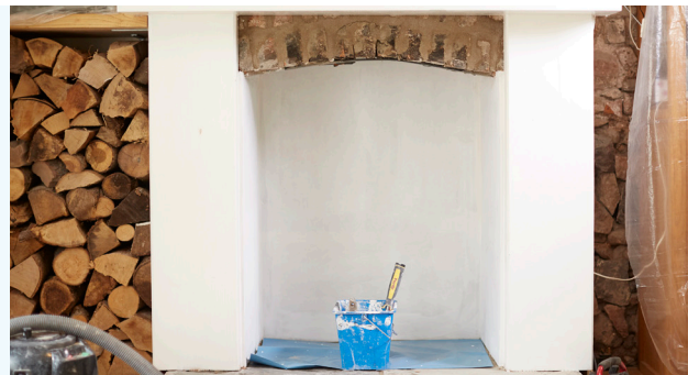
Allow 24 hours for the paint to dry.
