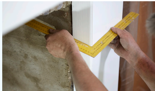
Using a right angle set square to check for uneven surfaces
