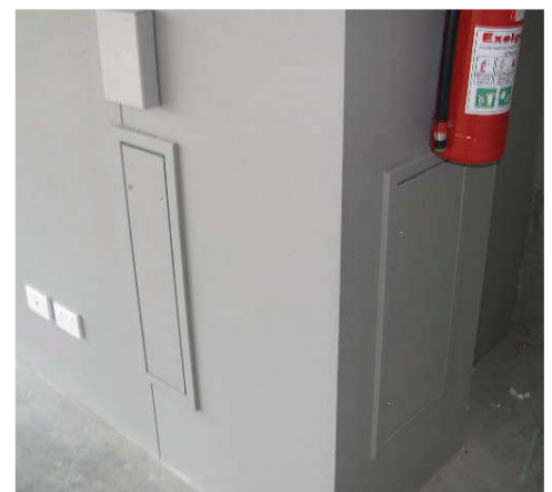
240 minute fire resistant PROMATECT®-S access panel (above) on the wall besides the railway track at the MRT station near People Park, Singapore.
