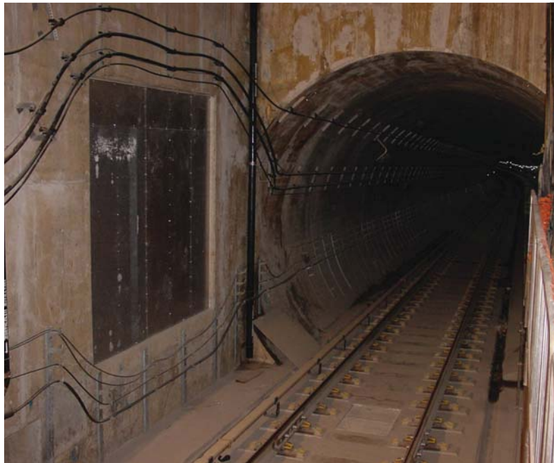
240 minute fire resistant PROMATECT®-S access panel (above) on the wall besides the railway track at the MRT station near People Park, Singapore.
