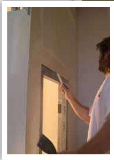
Plastering the board joints in partitions (left) and the junctions of wall and ceiling (above).
