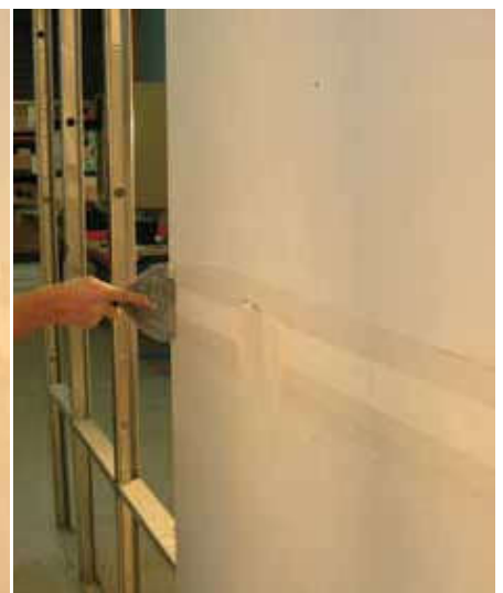
Final joint after finishing with trowel.
