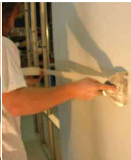
Apply subsequent covering of plaster compound to finish.
