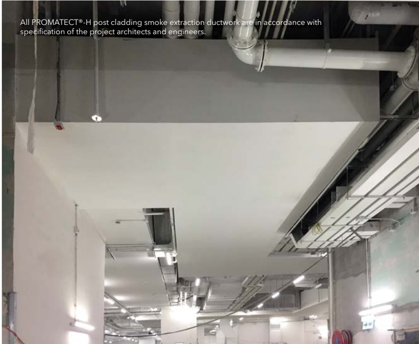
Some 3,000m 2 of 12mm thick PROMATECT®-H and 600m 2 of 20mm thick PROMATECT®-H are installed for the M&E services enclosure system throughout the project.
