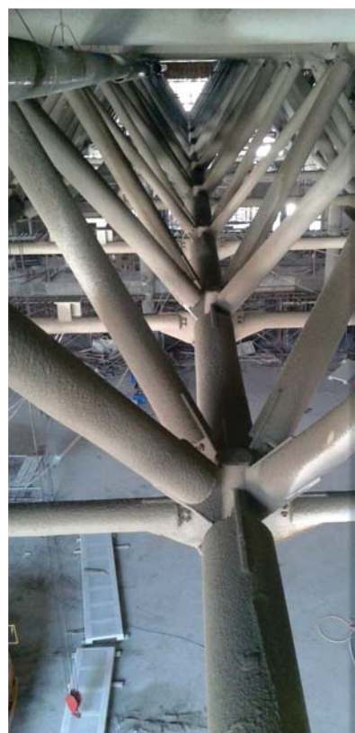
All pictures on this page Spray application areas of the main roof steel structures adjacent to the iconic roof at the exhibition hall.
