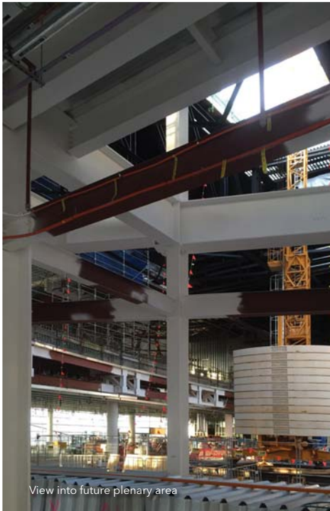
Main support steel of the convention floor
