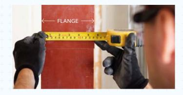
2 Mark up Flange Panel – Mark up VERMICULUX®-S board to fit flange plus 3-4mm.
