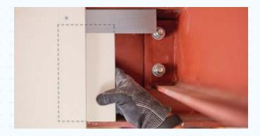
6 Flange Panel and Cover Strip - Measure, mark up and cut flange panel to fit between web panels, remember to pre-fix 120mm wide cover strip.
