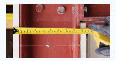
6 Mark up Web Panel – Mark up and cut VERMICULUX®-S board to the dimensions in step 5. (measure twice, cut once!)
