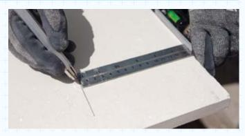
3 Cut Flange Panel – Cut boards using a hand saw with hardened teeth or a power circular saw in conjunction with tungsten carbide tipped blades, or a jigsaw. All cutting should be carried out in well ventilated spaces, using dust extractors.
