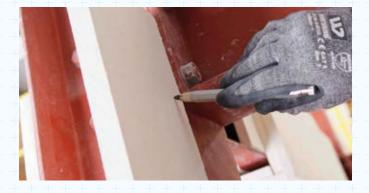
5 Measure for Web Panel – Measure the web of structural steel column plus the thickness of the VERMICULUX®-S flange panel. (20, 25, 30, 35, 40 or 50mm).
