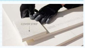
7 Fixing Flange Panel - Screw flange panels into position through the face of web panels at 200mm centres.
