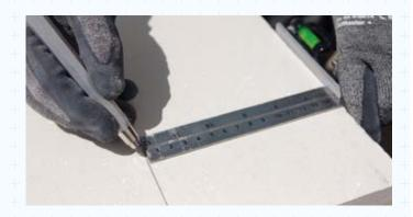
4 Fixing Web Panel - Fix web panels to steel angle using GTEC High Thread screws spaced at 200mm centres. Screws should be approximately half way down the angle.
