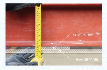
Measure Web Panel - Measure, mark up and cut VERMICULUX®-S boards to the dimensions in step 2, plus an additional 3-4mm.
