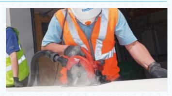
4 Column to Beam Junction – Mark up, cut and fit boards around junctions by butt jointing the square edges of VERMICULUX®-S.
