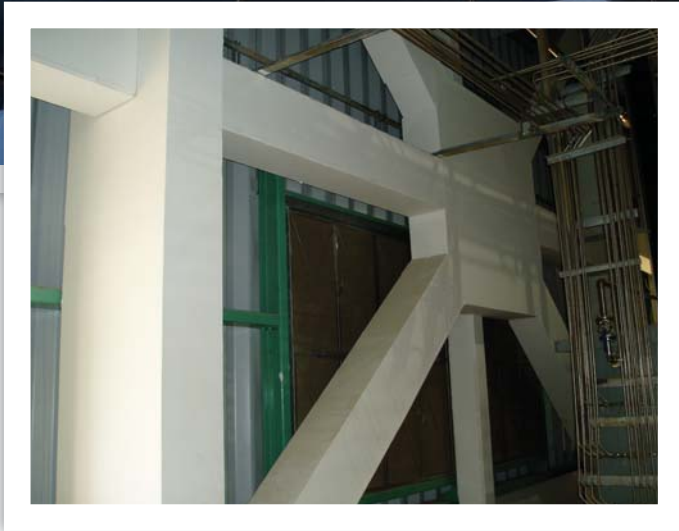
PROMATECT®-H structural steel column and beam cladding at the One Shelley Street office building (above) in Sydney, Australia and Tatan Power Point, Taiwan (left).
