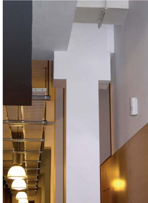
Cafco SPRAYFILM® WB3 structural steel coating at west side entrance of the Hong Kong Academy for Performing Arts and PROMATECT® 250 structural steel column claddings at the corridor of the Mallet Street residence apartments in Camperdown, New South Wales, Australia (right).
