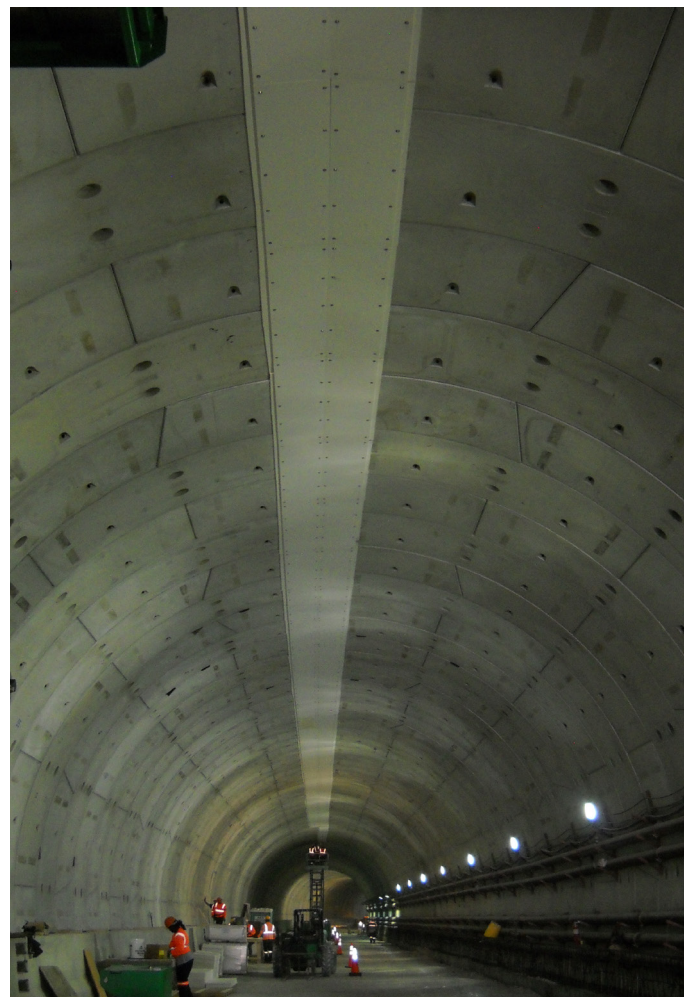
Initial centerline crown installation
