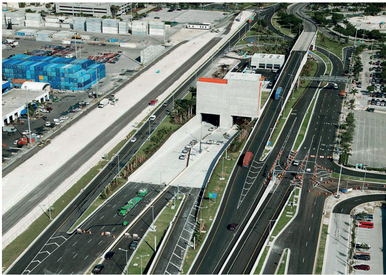
Port of Miami Tunnel Dodge Island Portal
