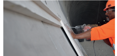
Installing 2 nd board to adjacent
