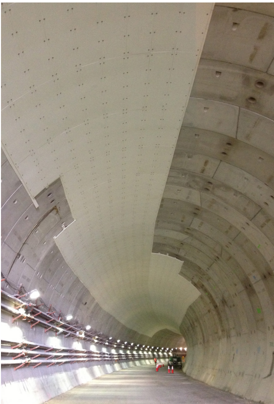
Installation of panels through curve
