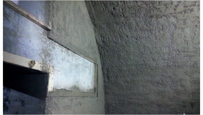
Port of Miami Tunnel PROMASPRAY®-F5 applied with a semi textured finish
