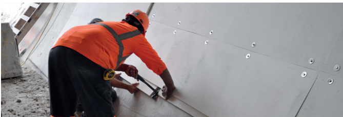
Slide backing strips into position
