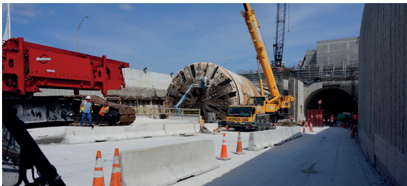
Port of Miami Tunnel Breakout on Watson Island Portal
