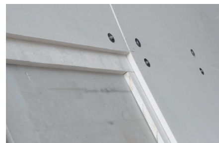
Port of Miami Tunnel facetted panel backer strip
