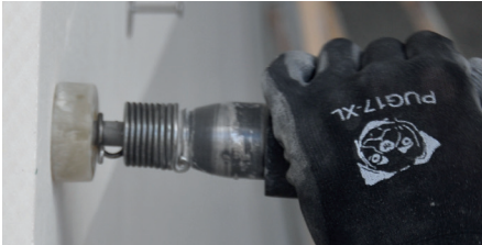
Setting anchor with pneumatic hammer
