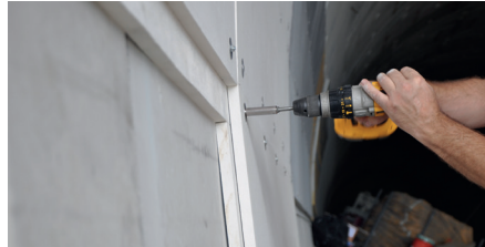
Tighten stainless steel nut with battery driver
